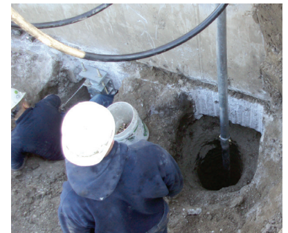
Helical pier extension advanced through pre-augered hole
