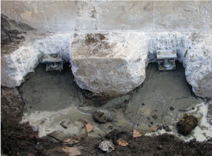
Completed pier with retrofit bracket; excavations filled with cement grout
