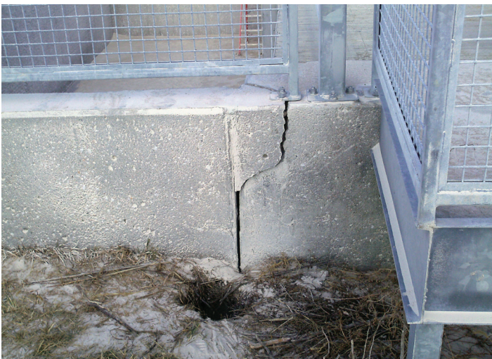
Fractured concrete
