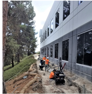
Piers being installed along the southeast wall
