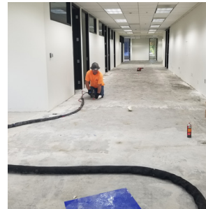
PolyLevel injection at interior floor slab
