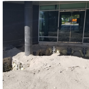
Push piers, anchors and PolyLevel installed at center patio area
