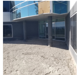
Pier locations backfilled and compacted at center patio area
