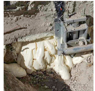
Underpinning bracket with integrated anchor and PolyLevel injection
