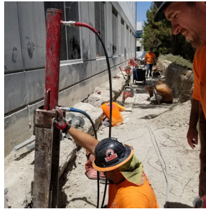
Installing push piers along the south wall
