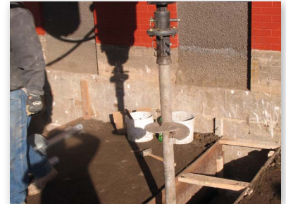
Preparing to install lead section - north deck
