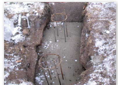
Grade beam poured - north deck
