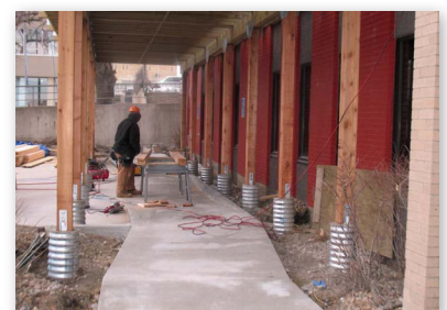
South deck supported by helical piles
