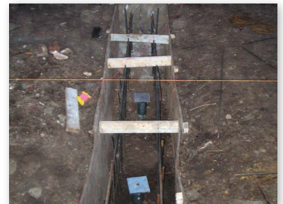
Tops of piles to be cast into grade beams
