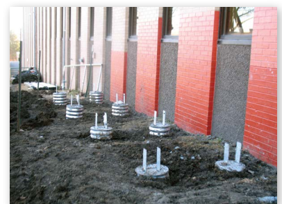
Concrete piers poured over the grade beams - north deck
