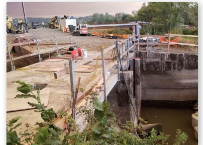
North side of culvert with temporary dam in place (on right)
