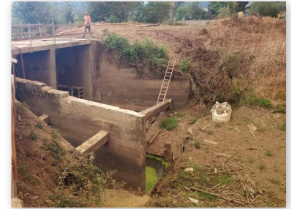
South side of culvert where stoplog wall would be constructed
