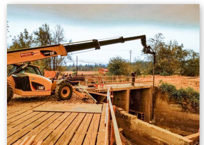
Reaching out for the last helical pile installation
