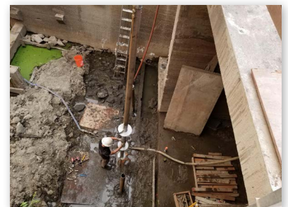
Installing a 10"-12"-14" helical lead section
