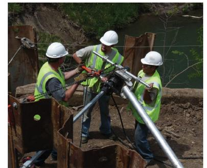
Tieback installation with handheld equipment
